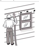
Although you may be able to rent the equipment for blowing insulation into your home's exterior walls, the job is very involved and is best handled by and experienced insulation contractor.
